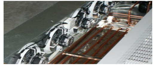
Vacuum dust and debris from the condenser unit and cooling fins
